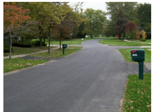
Repaving Meadowbrook Way (before: top, and after: bottom)
